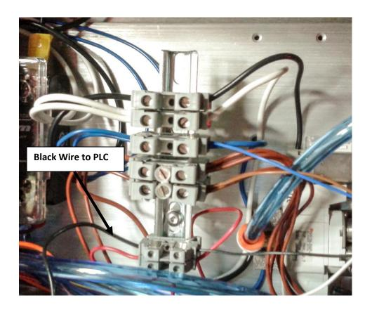
Run the Black Wire from the Grey Connector though the opening in the Side Panel to the PLC Expansion Card.
