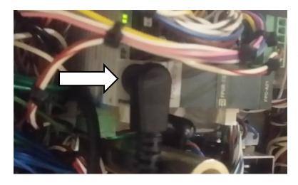
The Scale Board is to be connected directly to the PLC via the PLC programming port using a 5-pin Mini DIN plug.
